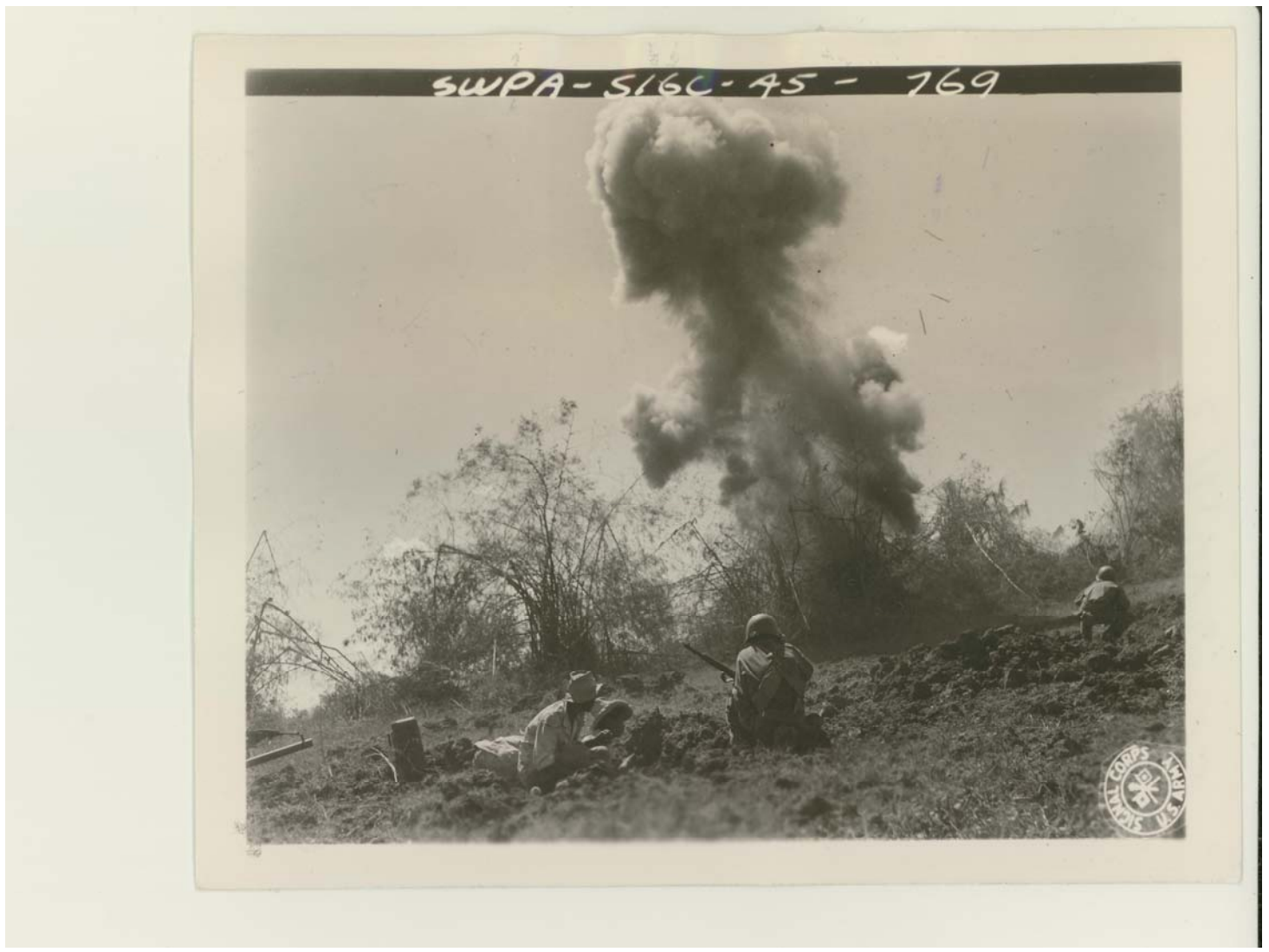
Demolition of a Japanese Pillbox
